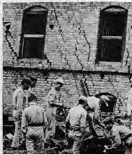
The 1988 Udaipur earthquake, (M=6.3) destroyed villages and towns in East Nepal such as Dharan, shown here.
